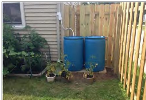
Dual rain barrels connected in series from the downspout diverter. Once barrels are full, rainwater continues down the downspout. Credit: Chagrin River Watershed Partners, Inc.
