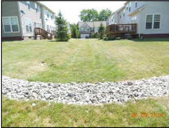
Well maintained vegetated infiltration swale with stone check dam. Credit: Chagrin River Watershed Partners, Inc.
