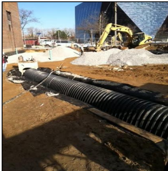
Installation of underground detention system within permeable parking lot at the Courtyard by Marriott hotel in Cleveland, Ohio. Credit: Northeast Ohio Regional Sewer District
